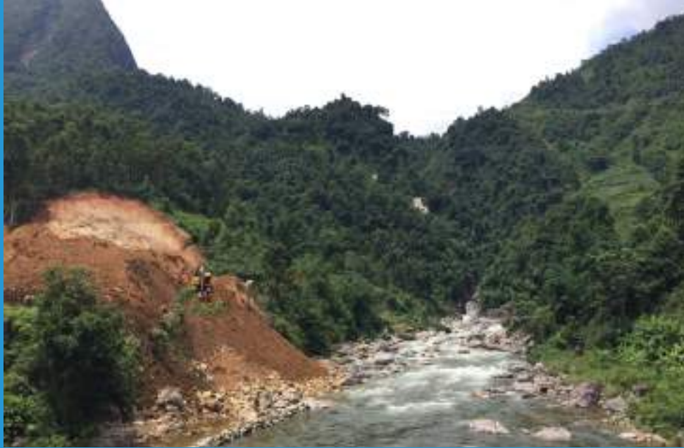
Hydropower is under construction
