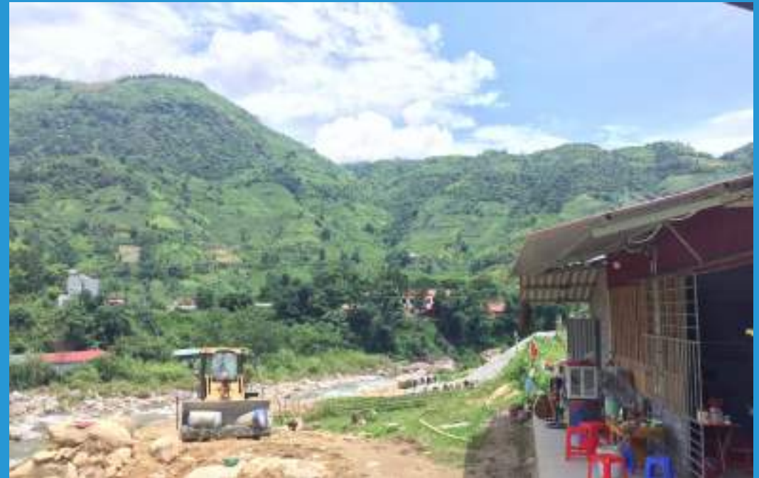
Hydropower is under construction
